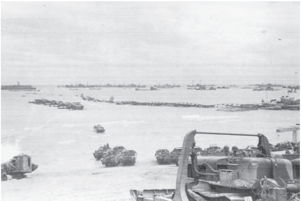
Figure 21: Mulberry Harbor at Omaha Beach. General Huebner's scrapbook, MRC
